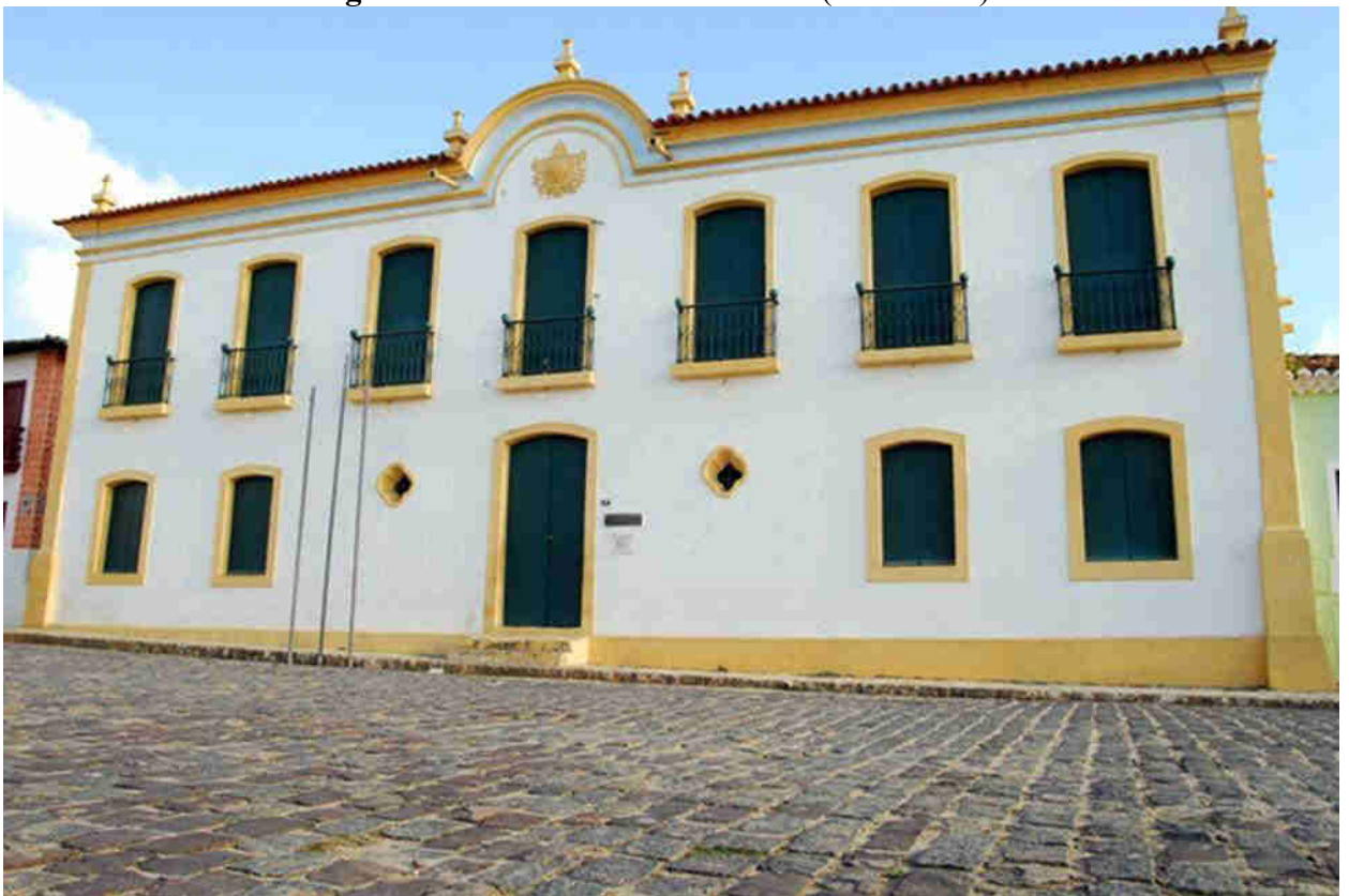
Figure 2: MHS after last restoration (2007/2009)
