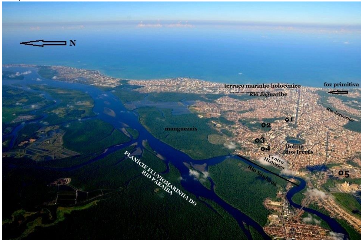
Figure 2- Aerial view of the Paraíba River estuary and the municipality of João Pessoa, with the location of the Sanhauá fault, the Jaguaribe River and its primitive mouth before the Holocenic sedimentation, in addition to the Dolina dos Irerês and the fountains of the Historic Center (1- Bica Maria Feia; 2- Tambiá; 3- Santo Antônio; 4- Miracles and; 5 - Cacimba do Povo). The dashed line shows the inactive cliffs that delimit the boards (to the west) of the Holocene marine terrace (to the east).
