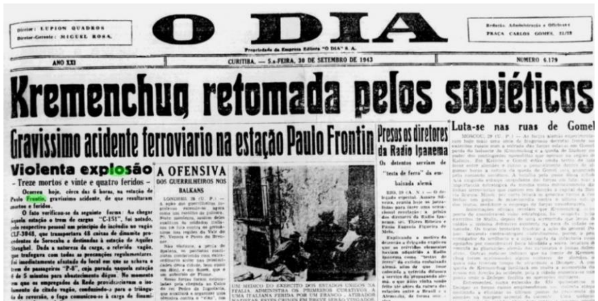
Image 2 – Explosion (thirteen dead and twenty-four injured).
